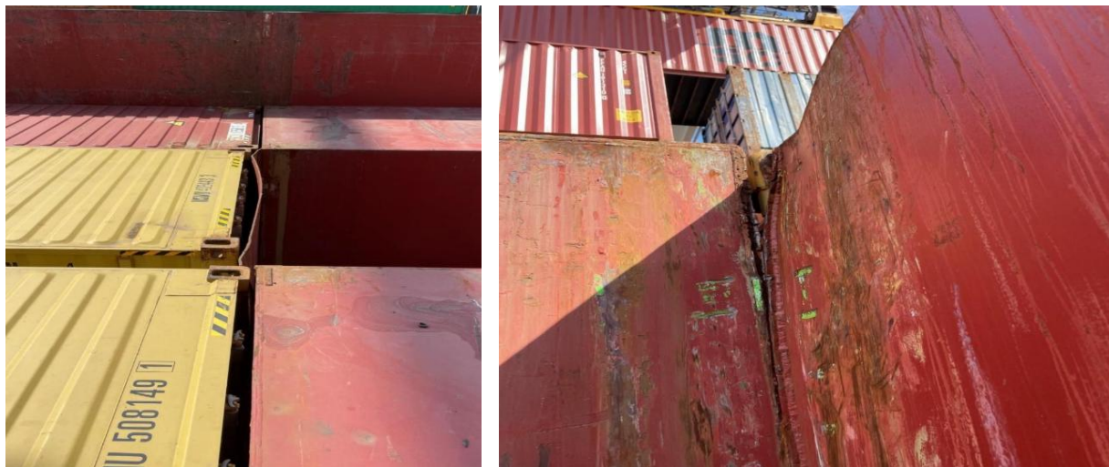
12 | Damages on the protection bulkhead on the Alphenaar
